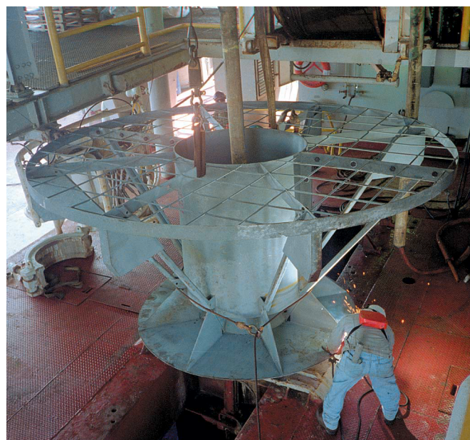
ROV platform being assembled in the moonpool for free-fall deployment to finish the CORK installation in the reentry cone.
